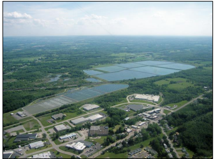
The City Wastewater Treatment Plant was built in 1990 and can treat up to 5.5 million gallons per day of influent.
